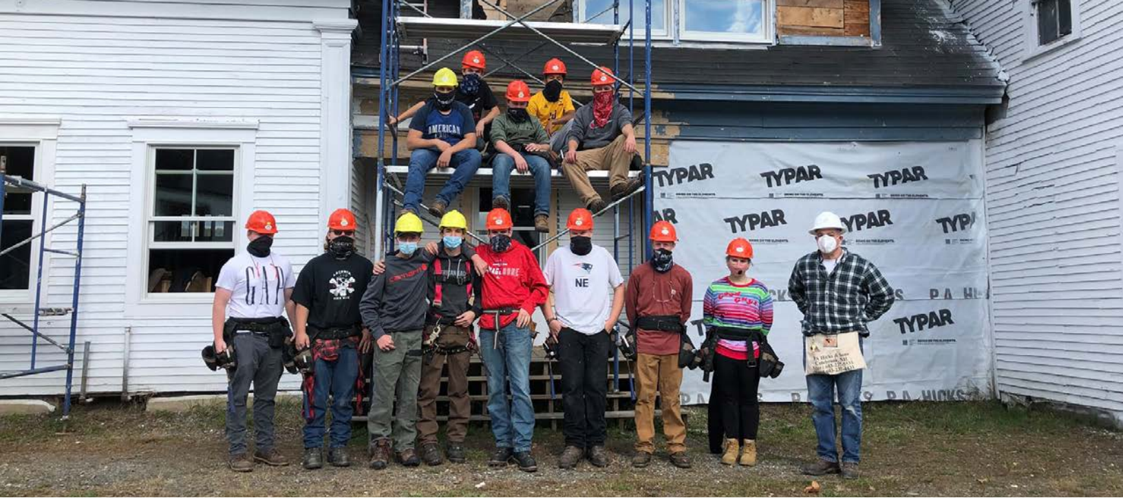
Canaan Memorial High School Building Construction and Restoration Carpentry program, Colebrook, NH. Photo: New Hampshire Preservation Alliance
