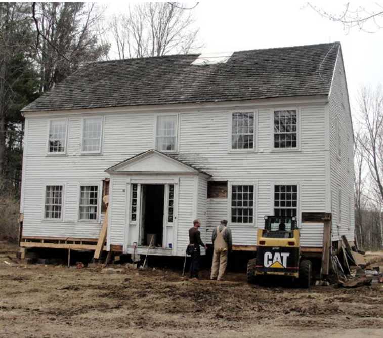
Foundation and sill work. Photo: New Hampshire Preservation Alliance
