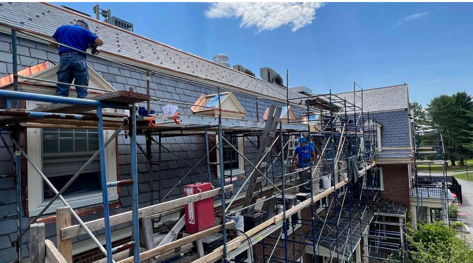
Slate roof restoration by The Heritage Company, Colby College, Waterville, ME. Photo: Maine Preservation
