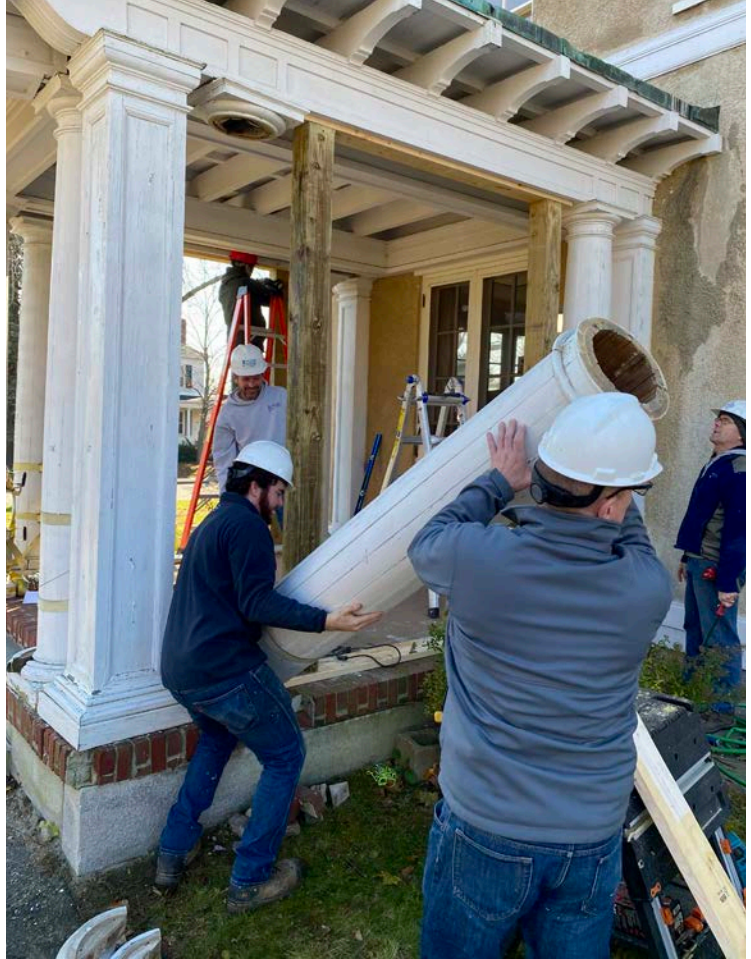
Porch restoration at the First Amendment Museum, Augusta, ME. Photo: Maine Preservation.
