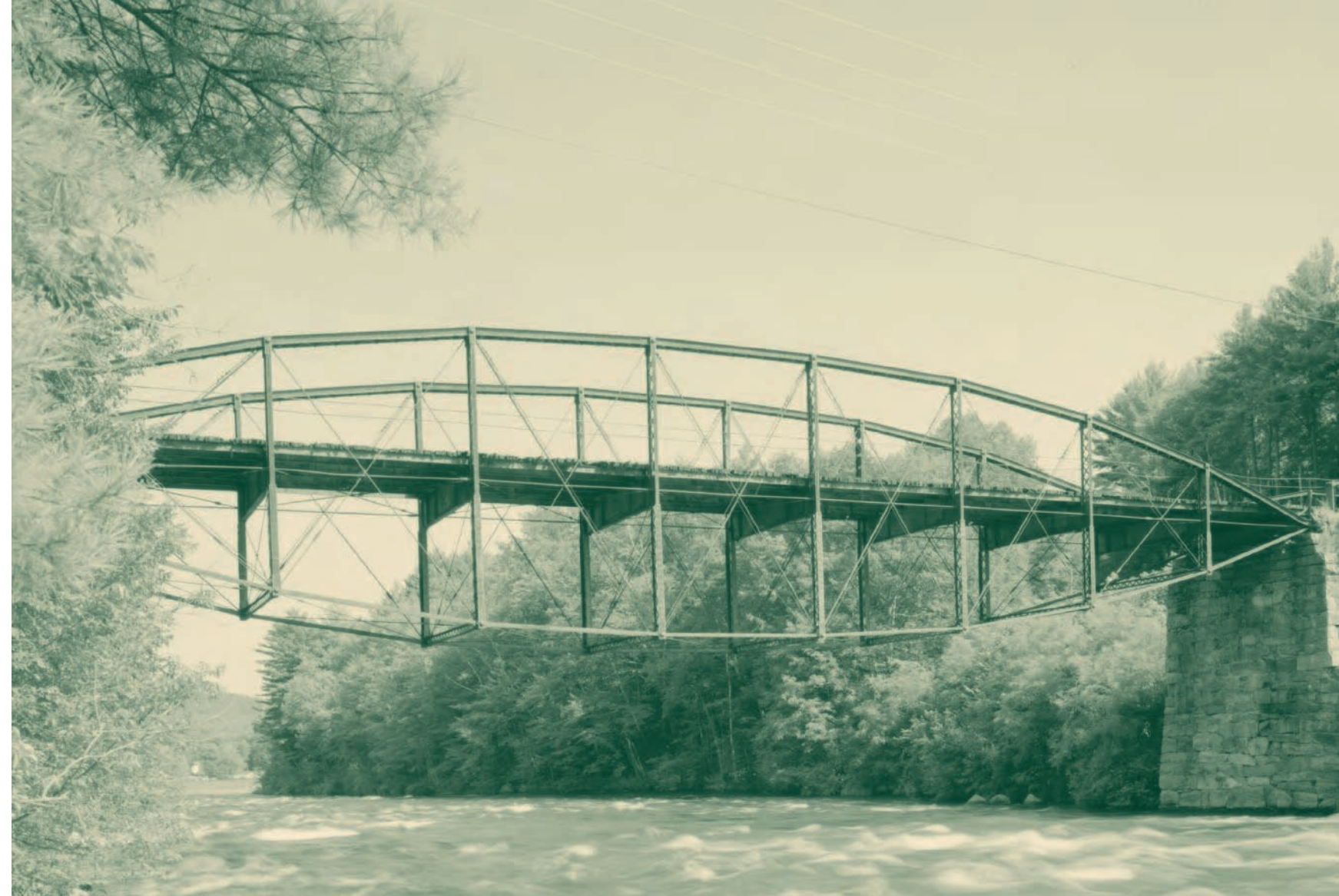
Upstream view looking southeast from river level, prior to rehabilitation.
