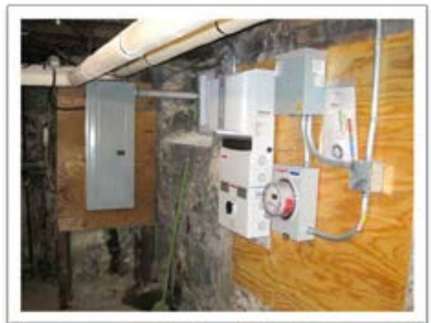
18. Balance of System Wall Photos – A pull-back photo showing the entire balance-of-systems equipment wall (may need multiple photos).
