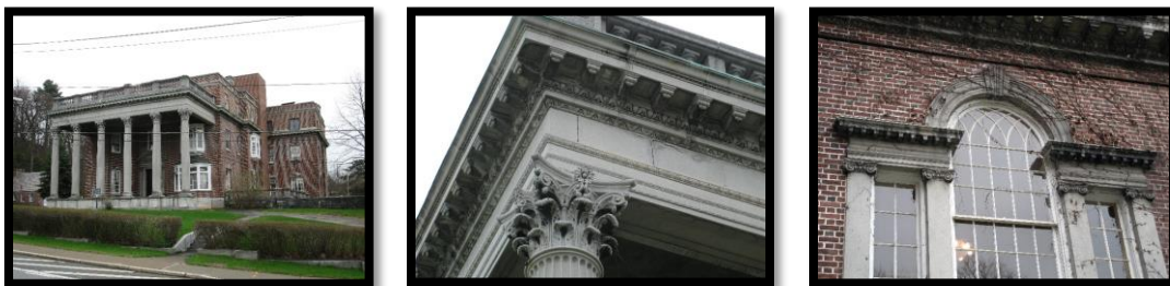
Exterior images of Amsterdam City Hall (City of Amsterdam).
