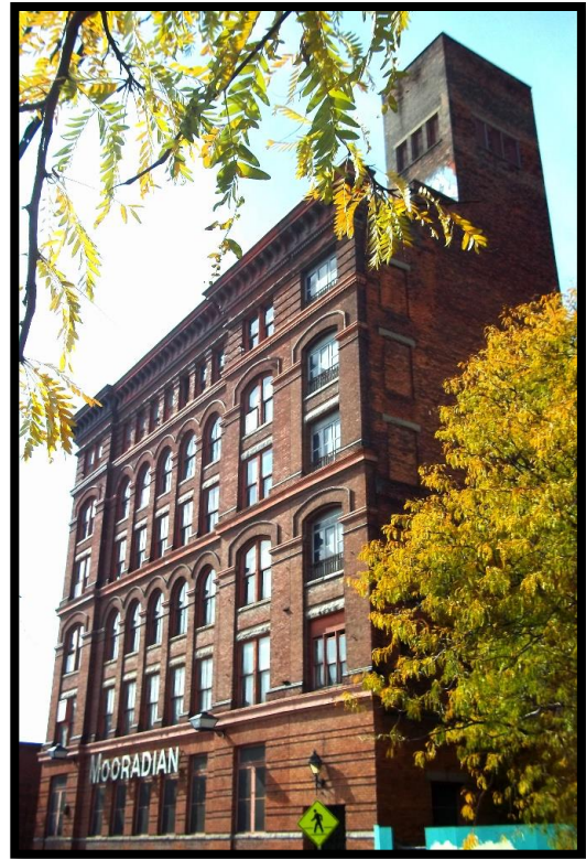
Mooradian Building, River Street, Troy (M. Lopez).
